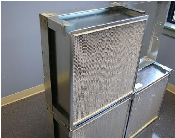
Figure 5: Filter placed inside of frame.
