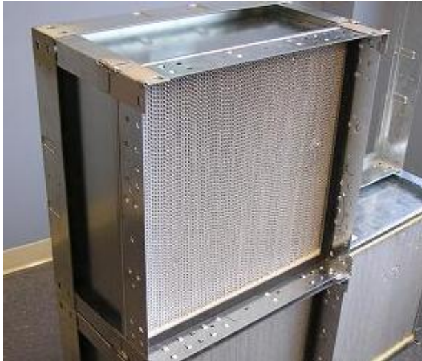
Figure 10: Properly installed HEPA filter.
