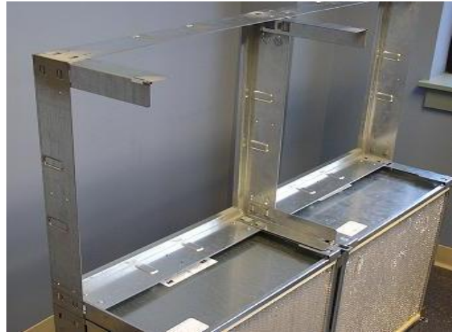
Figure 3: Frame with leg extensions installed
