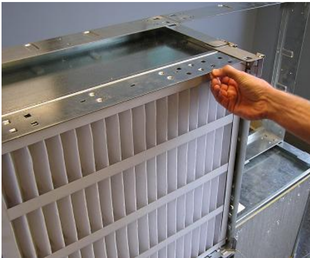
Figure 11: Installation of prefilter into frame.
