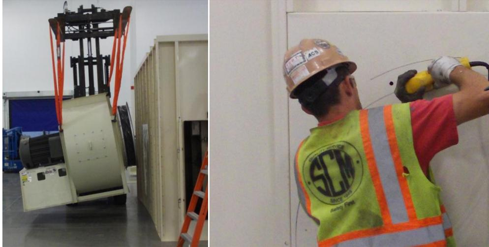
**NOTE: BE SURE the fan is in the exact position it will be in when in operation, whether mounted on the floor or on a stand. Shim and align the fan in the proper location. The fan can be either mounted directly to the Fan Panel or to the Fan Panel via a flexible connector, spool piece or transition. If vibration isolators are supplied, be sure to install them on the fan before installation**
