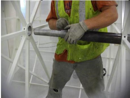
NOTE: Be sure the drive end (Keyed end) of the Shaft (Item 14) is facing the drive end, whether the drive end is in the front or the back of the Drum Filter.
