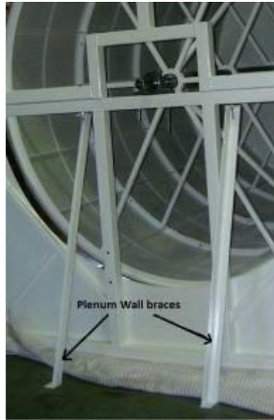
4.7. If the plenum wall is split you will have to fill the gap in the angle rings between the top and bottom plenum wall panels with body filler (supplied by Ibis). Allow filler to dry and then sand smooth. This will allow the primary seal to slide smoothly around the angle ring
